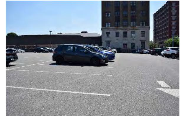
Stormwater runoff from this expansive parking lot drains to multiple catch basins on the north, south, and west ends. Parking spaces on the far edges of the parking lot can be retrofitted with porous asphalt to allow for the capture and infiltration of stormwater runoff from a majority of the parking lot. A preliminary soil assessment suggests that more soil testing would be required before determining the soil's suitability for green infrastructure.
