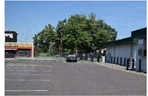
Stormwater currently drains to multiple catch basins in the parking lot, and the trailer's downspouts discharge onto the pavement. Porous asphalt can be installed adjacent to the trailer building to capture a portion of the runoff from the roof. A preliminary soil assessment suggests that more soil testing would be required before determining the soil's suitability for green infrastructure.
