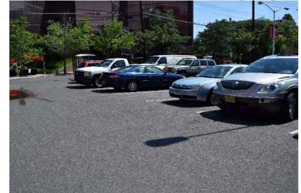
Stormwater drains to catch basins in the center of the parking lot and pools in some areas. Porous asphalt can be installed in the parking spaces to capture, treat, and infiltrate stormwater runoff. A preliminary soil assessment suggests that more soil testing would be required before determining the soil's suitability for green infrastructure.
