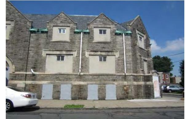
There are multiple downspouts on the east side of the church that direct water onto the sidewalk. Downspout planters can be installed on the sidewalk to capture stormwater from the downspouts. At the front of the church, a rain garden can be installed to capture runoff from a portion of the building by redirecting downspouts into it. A preliminary soil assessment suggests that more soil testing would be required before determining the soil's suitability for green infrastructure.
