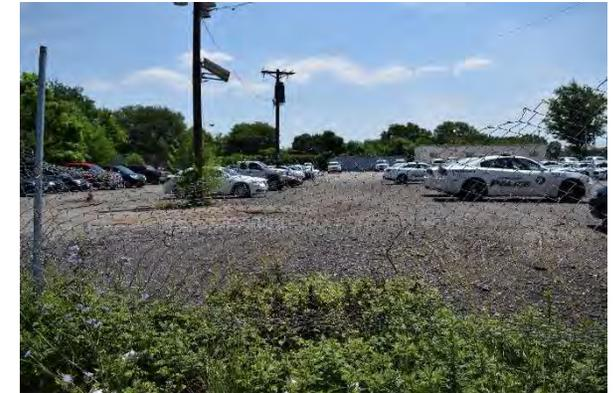
This police department station has a large compacted gravel parking lot that causes large volumes of stormwater runoff. Porous asphalt can be installed in the rows of parking spaces to capture runoff and improve stormwater infiltration. A preliminary soil assessment suggests that more soil testing would be required before determining the soil's suitability for green infrastructure.
