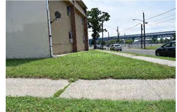
The apartments have disconnected downspouts directed towards the road on the west side of the buildings. Several rain gardens can be installed in the existing grassed areas to capture, treat, and infiltrate rooftop runoff. This garden can add to the aesthetic of the site and create wildlife habitat while also managing stormwater runoff. A preliminary soil assessment suggests that more soil testing would be required before determining the soil's suitability for green infrastructure.
