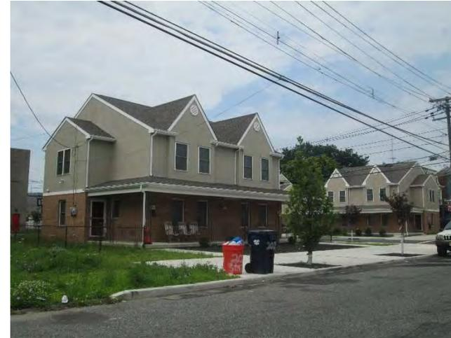
The existing downspouts can be disconnected and redirected into rain gardens in the grassed area at the front of the home to capture, treat, and infiltrate water from the rooftop. There are a series of homes with a similar set up throughout North Camden that could also receive rain gardens. A preliminary soil assessment suggests that more soil testing would be required before determining the soil's suitability for green infrastructure.
