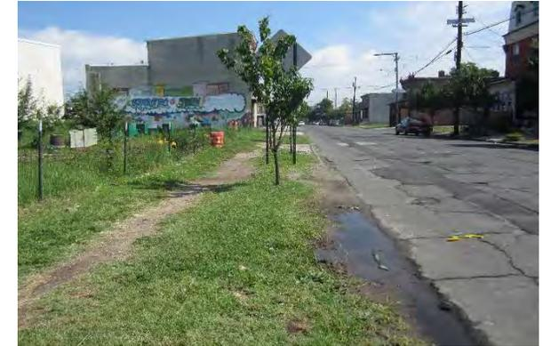
Stormwater sits on the side of the road next to the garden where there is no curb. A stormwater planter can be installed along this area to capture, treat, and infiltrate stormwater from the road. A cistern can be installed to capture runoff from the adjacent shed for reuse in watering the garden. A preliminary soil assessment suggests that more soil testing would be required before determining the soil's suitability for green infrastructure.
