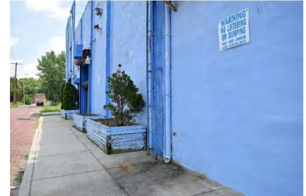
Some of the downspouts are in disrepair and currently direct stormwater onto the sidewalk. Some of these downspouts can be redirected to the rear of the building to capture, treat, and infiltrate roof runoff. Additionally, downspouts could be redirected into the existing planter boxes to treat a portion of their runoff. A preliminary soil assessment suggests that more soil testing would be required before determining the soil's suitability for green infrastructure.
