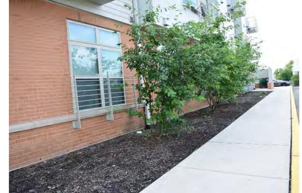
There are multiple existing raised bed gardens which could benefit from a cistern on site. An existing downspout can be disconnected into the cistern to harvest stormwater from the rooftop. Along the north and west ends of the building downspouts could be disconnected rain gardens that could be incorporated into the existing landscaping. A preliminary soil assessment suggests that more soil testing would be required before determining the soil's suitability for green infrastructure.
